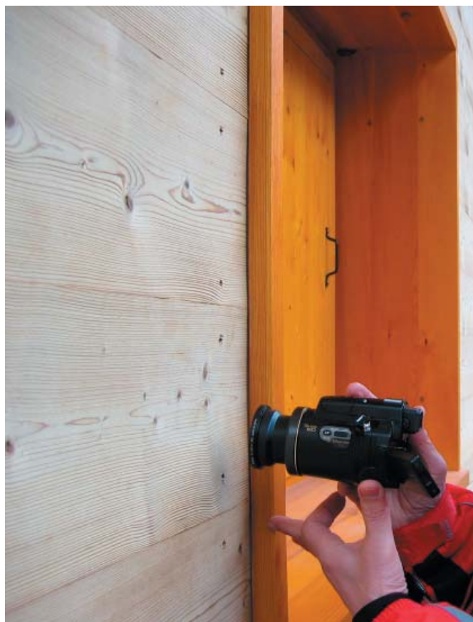
Close inspection of heat treated spruce cladding.
